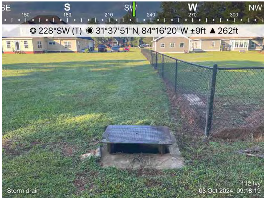
Figure 8 – Inlet on side of 112 and 106 Ivy Lane
